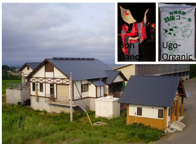
Overview of Urine Treatment Plant
